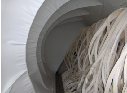
Drainage loops inside the tank
